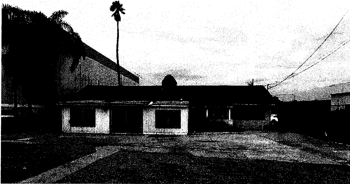
Figure 4 View of Primary (East) Façade, 13551 Harbor Boulevard
