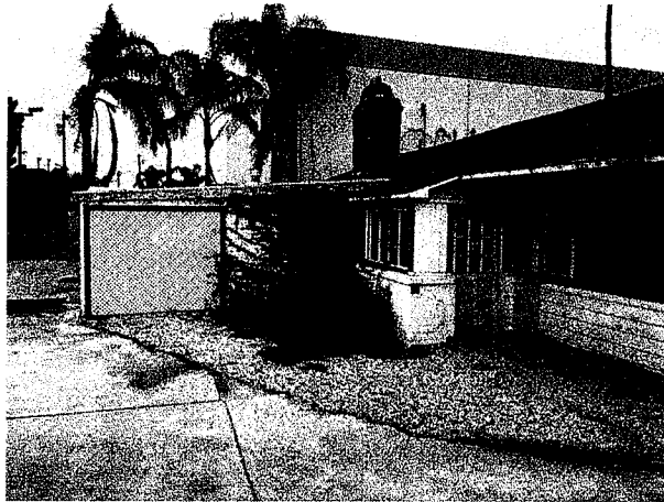
View of East Façade and Entrance
