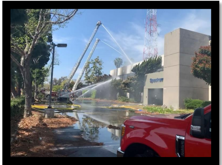
Structure fire in Garden Grove on 4/4/22.
