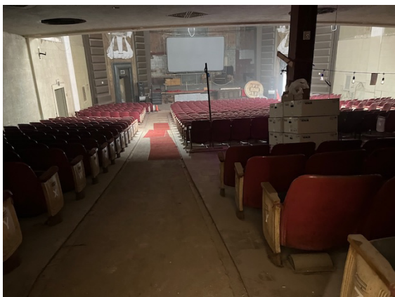
Auditorium interior. The somewhat misty look in the photo is due to construction dust
