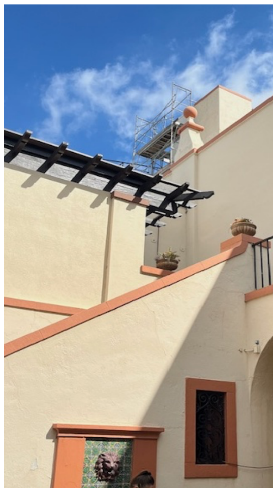
Scaffolding is visible along the roofline
