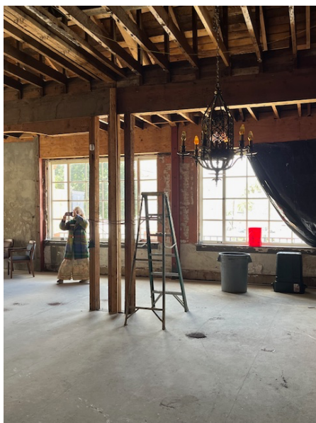
More storage above the lobby and entrance area
