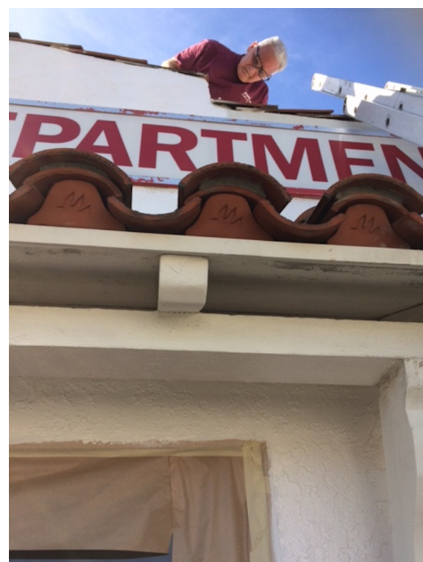
Jeff Harlan at work on the roof
